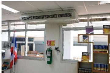
Air-Conditioned Building (ARU, Thailand)
