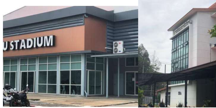
4. Buildings with transparent glass windows (Ubon Ratchathani Rajabhat University, Thailand)
