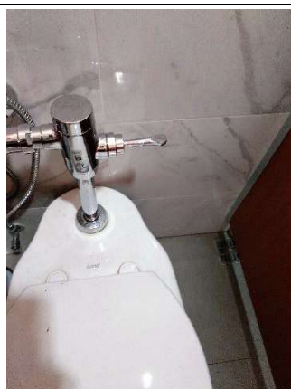
Efficient toilet flushes installed in new building
