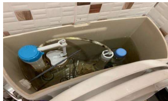
Low-cost technique by replacing a water bottle inside the water tank, helping reduce the water use by 25%
